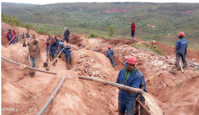
Mineral washing process through sluices
